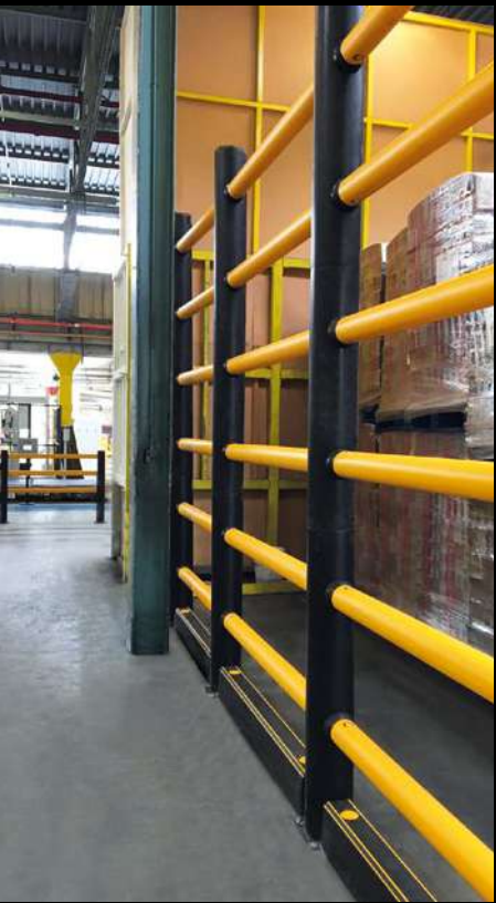
iFlex Topple Barrier protecting pedestrians from stacked bulk goods.
