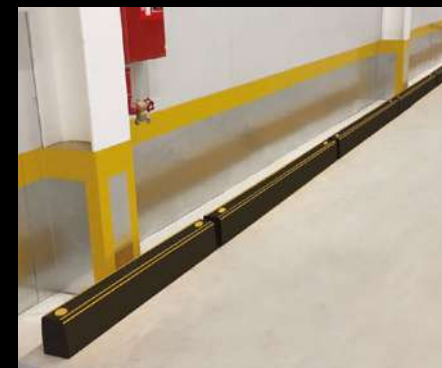
ForkGuard protecting walls at ground level in a distribution facility.
