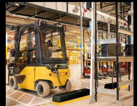
Step Guard protecting EV charging station.
